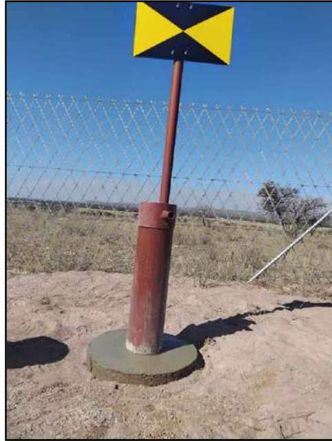
Photo 2: MON01 after complete installation
